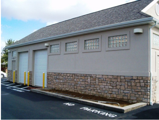
New Boiler Building
