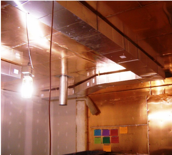
Pictures of Room Under Construction with Copper RF Shielding shown prior to cover up with insulation & drywall.
