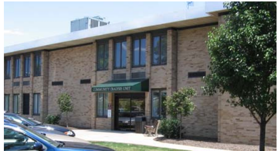
Mercy Hospital Community Dialysis: A renovation of approximately 6200 Sq. Ft. to upgrade an existing dialysis center and improve on temperature and humidity conditions.
