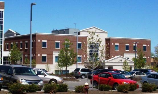
Alliance Hospital Medical Office Building: A new nominal 50,000 Sq. Ft. Medical Office Building with General Medical Offices, a Dialysis Suite, an Endoscopy Center, and Administrative Offices.
