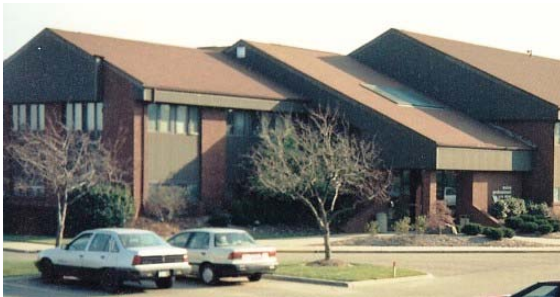
Aultman Medical Office Building: A Mechanical System Upgrade replacement of a nominal 9,200 Sq. Ft. area (1 st Floor) within an existing facility. Upgrade faced many space and zoning challenges
