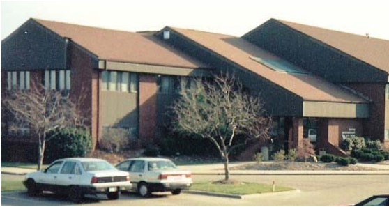
Aultman Medical Office Building: A Mechanical System Upgrade replacement of a nominal 9,200 Sq. Ft. area (1 st Floor) within an existing facility. Upgrade faced many space and zoning challenges
